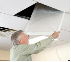
6. Position diverter on top of suspended ceiling under the leak. Run the hose to a drain or collection container.
