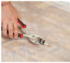
Slide clamps over the barbed fitting and pinch together with pliers to secure the clamp onto the hose and fitting.
